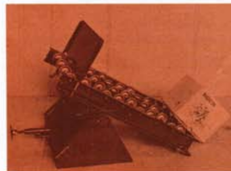
On this special Pack Stand cartons are first filled (top picture) then stand is tripped and carton proceeds along conveyor to warehouse or shipping.
